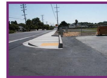
ments, 14 curb ramps, a sidewalk bypass around a joint utility pole, and five driveway conformers were installed along the south side of Pacifica Avenue (between Wharf Drive and Port Chicago Highway). This project brings this segment of Pacifica Avenue into compliance with the Americans with Disabilities Act (ADA).
